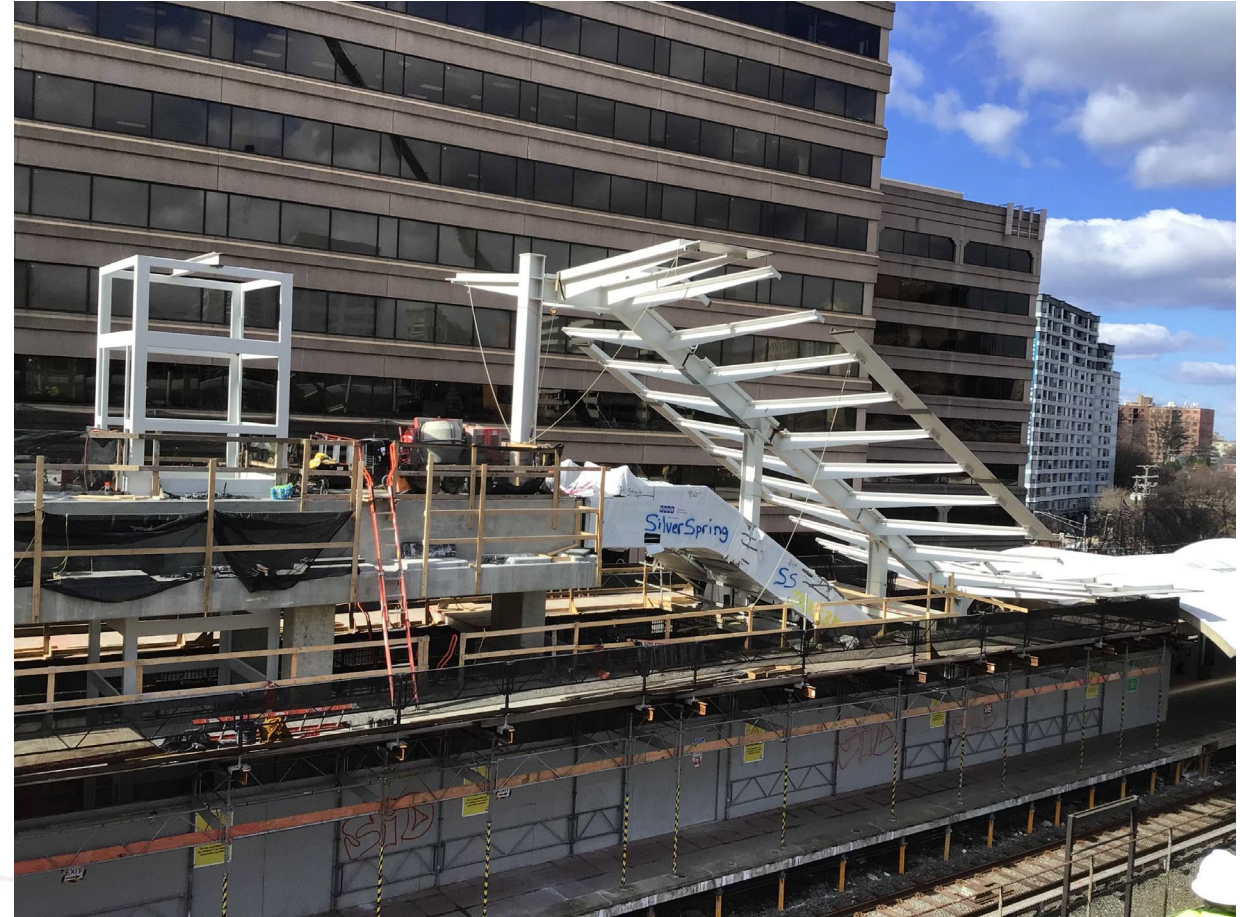
Metro Mezzanine Escalator and Canopy Frame installation at the Silver Spring Transit Center (Feb. 2025)
