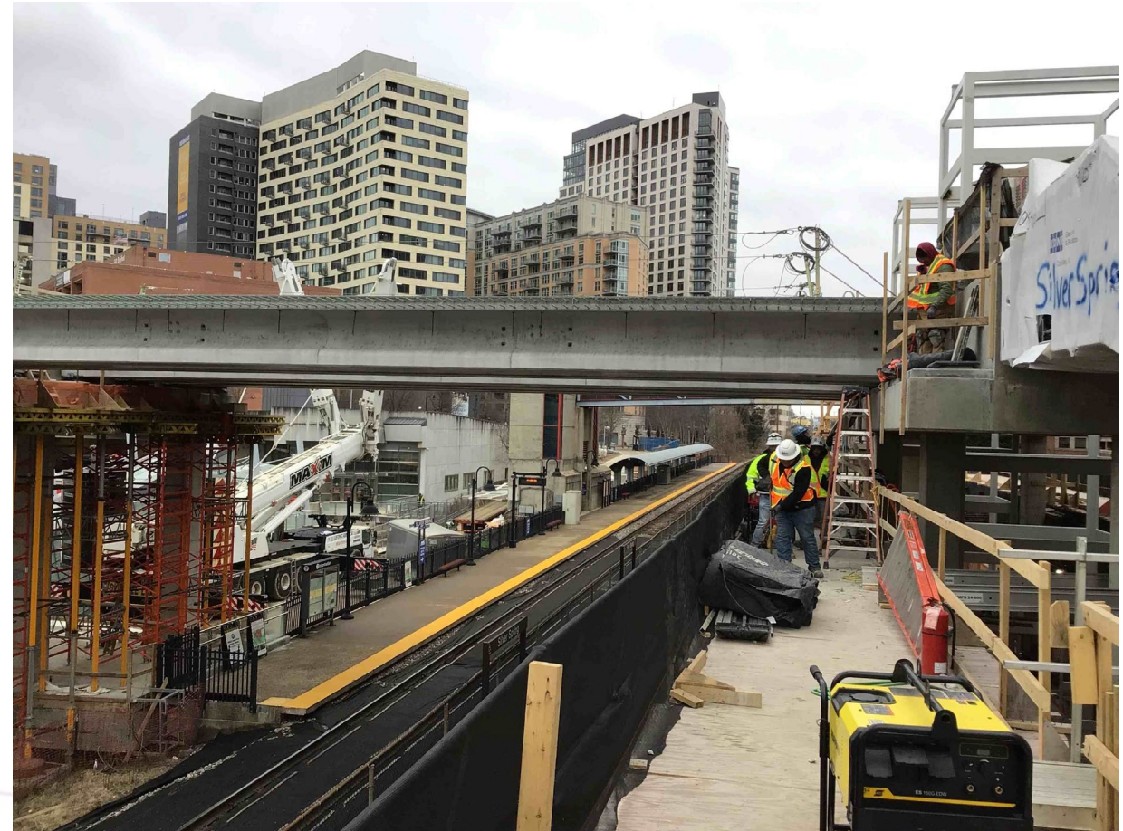
Mezzanine Girder Installation across Metro tracks at the Silver Spring Transit Center (Mar. 2025)
