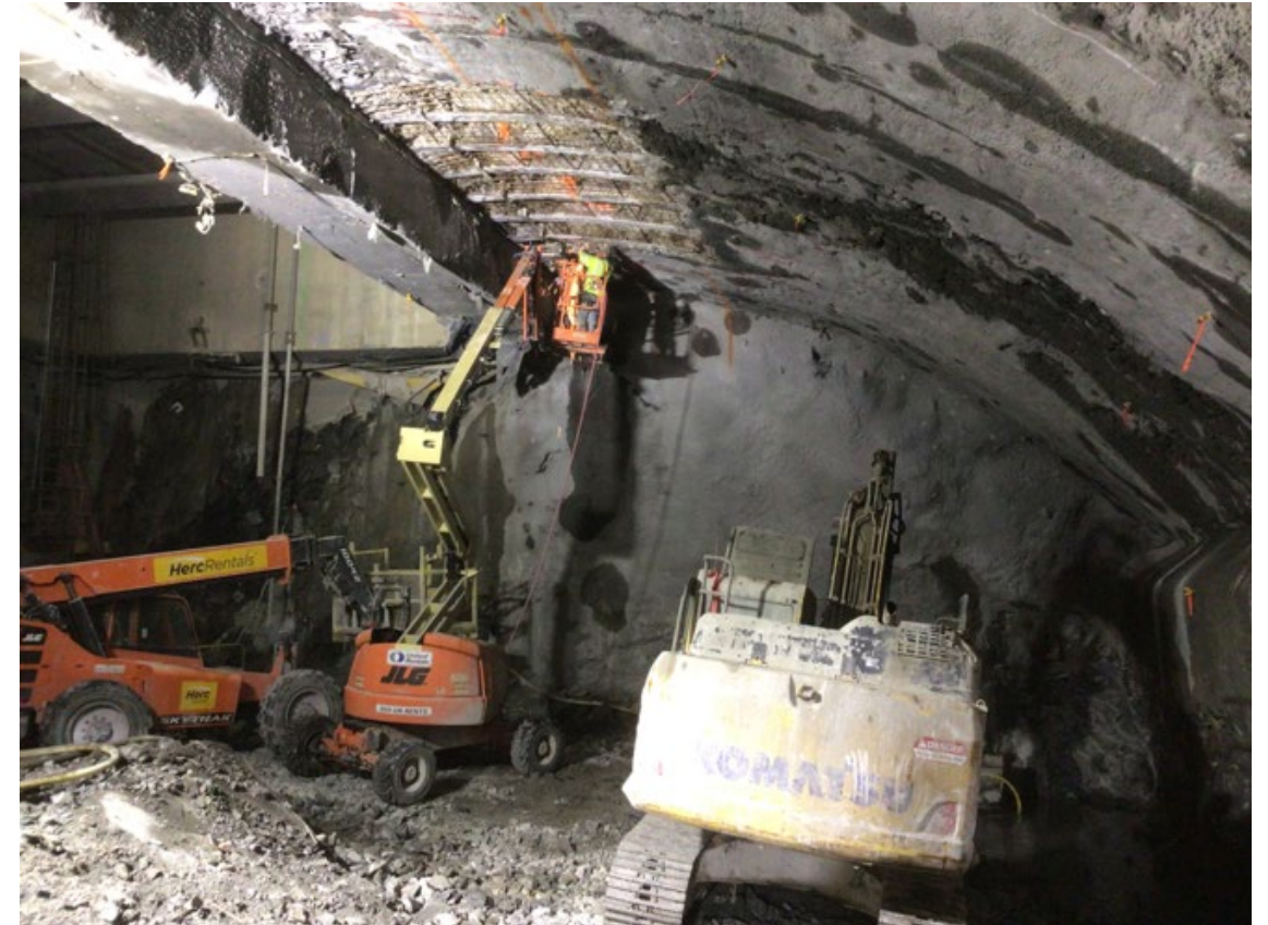
Construction of Bethesda South Station Entrance underway. Cavern arch concrete completed.
