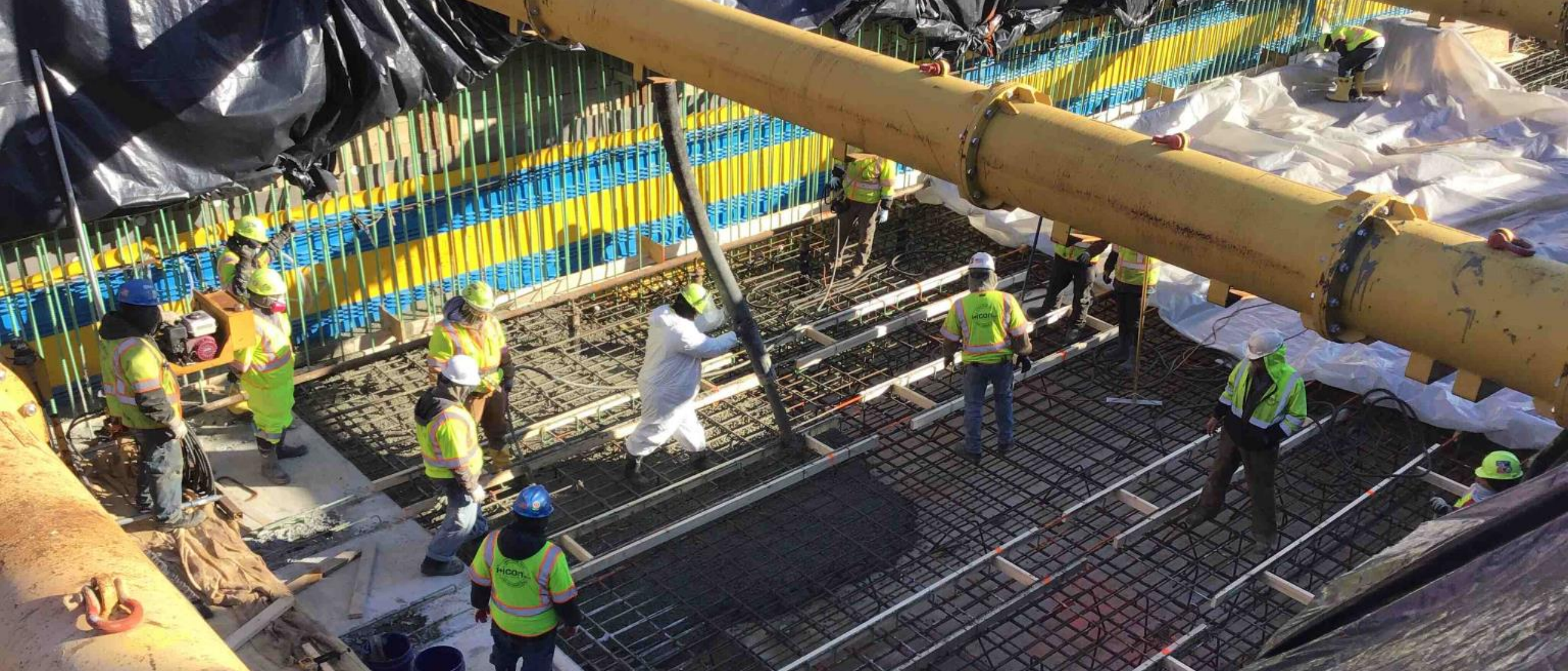
Long Branch: East Cut & Cover Track Slab Concrete Placement on Arliss Street
