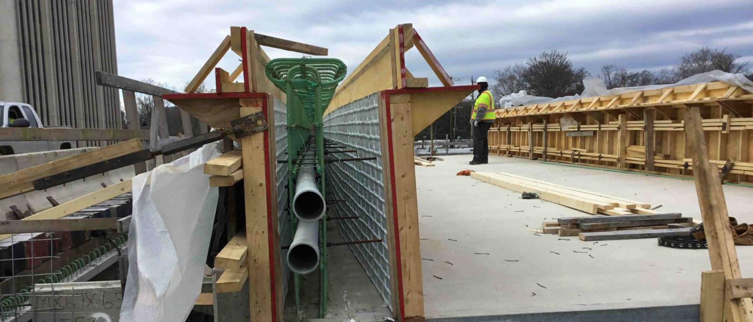
Bethesda: Parapet Formwork at Chevy Chase Lakes Terrace
